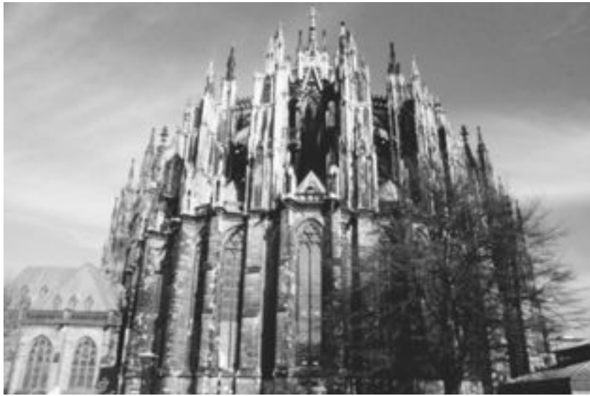
Figure 8.5. The outside of the Gothic choir of Cologne Cathedral highlights the flying buttresses reaching toward heaven.
